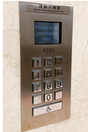
FIGURE 1.1: A typical keypad used to enter destination floors in a destination dispatch regime [15].
