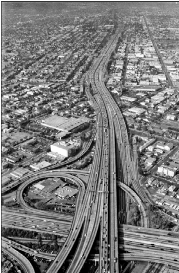
Figure 3: The freeways and urban sprawl that cover the landscape of much of Los Angeles.
