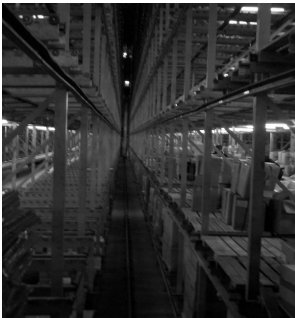
Figure 3: The fixed rail down an aisle on which a single crane operates.
