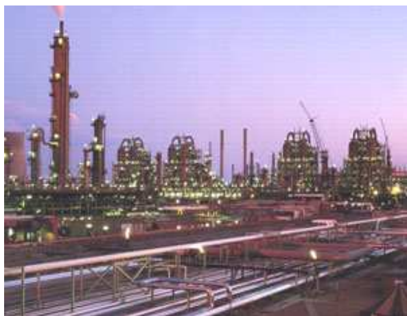
Figure 1: The Sasol Secunda Plant.
